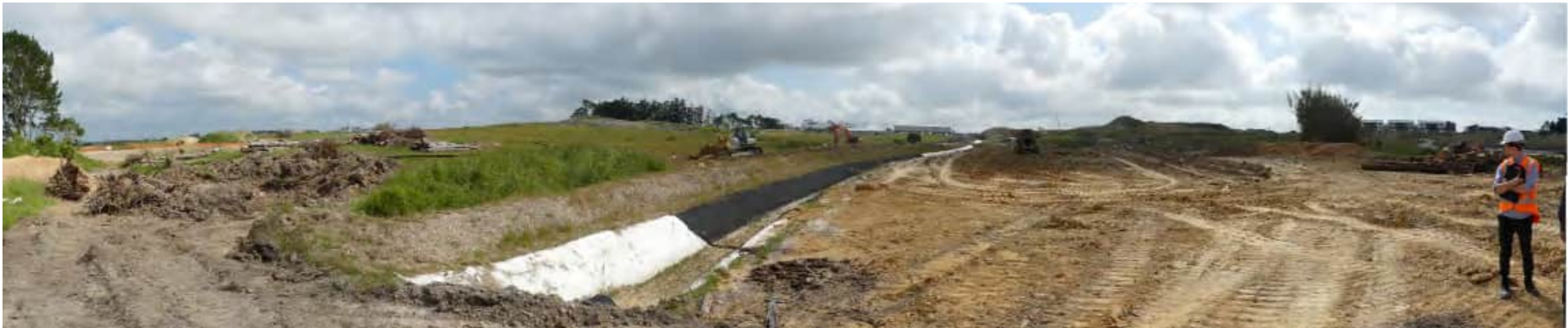
Viewpoint Photograph 03. Looking north over constructed stormwater - towards Dunlop Road. 50mm focal length. Standing eye level.
